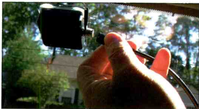
Attaching the coax to the inside coupling box is easy if you've done your homework and not made the installation a rush job. Note the short braid/strap coming out from the headliner and attached to the box.
