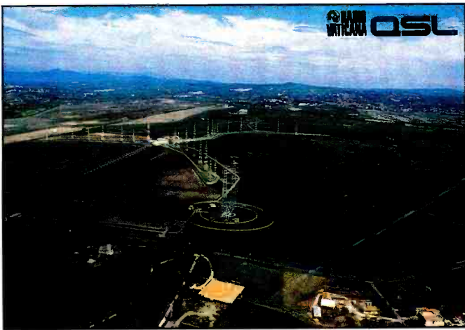
This is the Vatican Radio transmitter site at Santa Maria di Galeria. (Thanks Robert Charlton)
